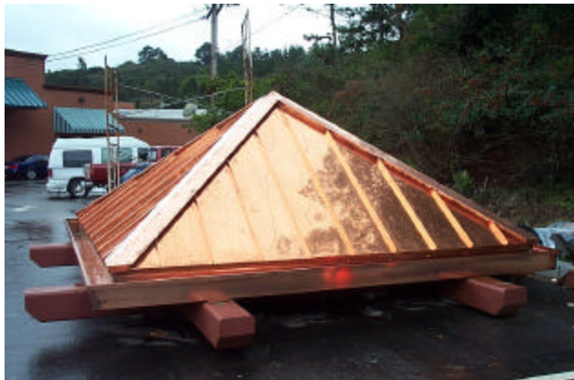
Copper roof section, prior to installation
