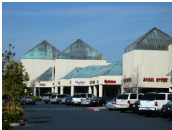
Copper roof, Redwood Shores California
