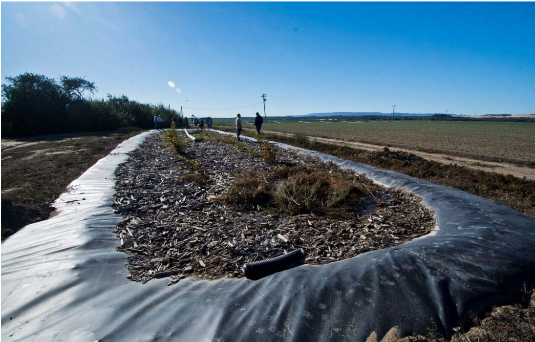
Figure 2. Bioreactor adjacent to Little Oso Flaco Lake.
