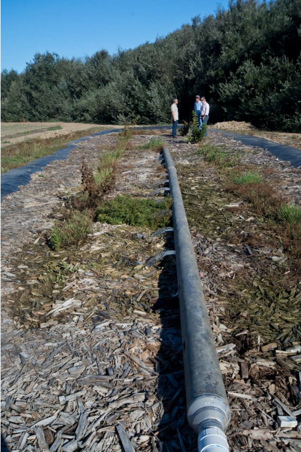
Figure 1. Bioreactor adjacent to Little Oso Flaco Lake with pump on and water flowing into bioreactor
