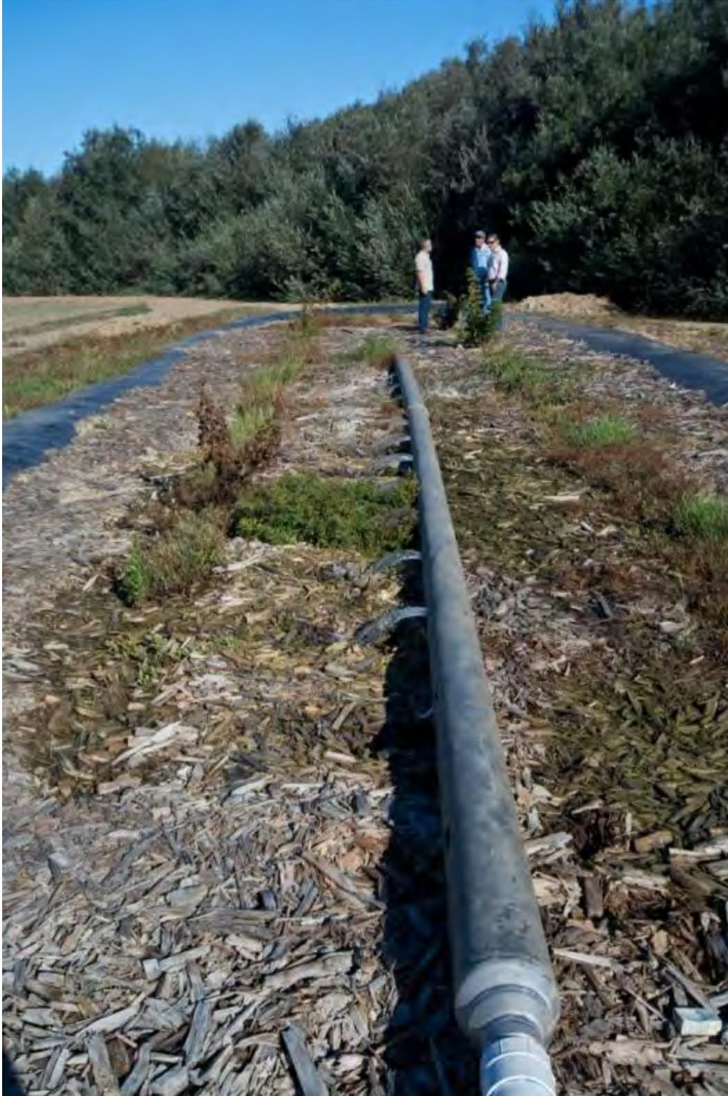
Figure 3. Bioreactor adjacent to Little Oso Flaco Lake with pump on and water flowing into bioreactor.
