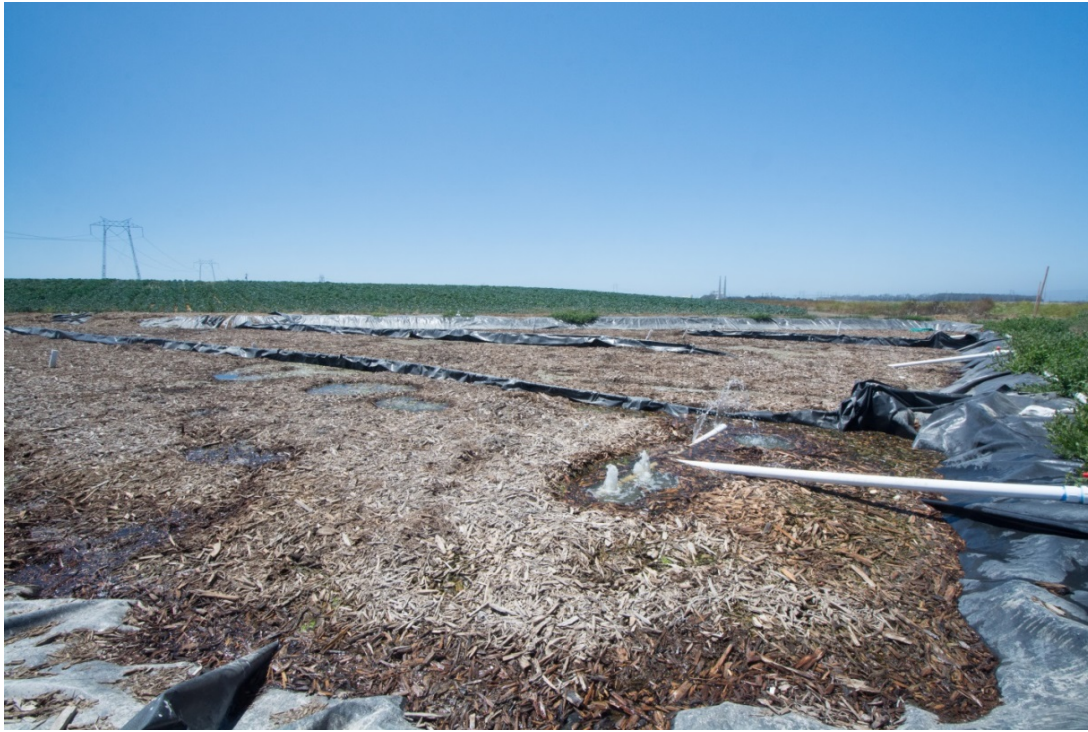
Fig. 1. Woodchip bioreactor, with inlet in foreground, on Sea Mist Farms in Castroville, CA. July 2016.
