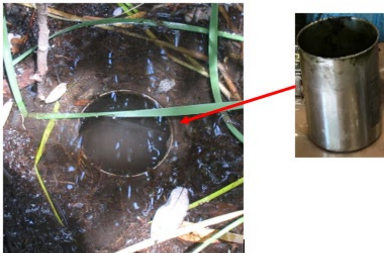
Figure 5: Stainless steel sediment trap installed in a stream bed
