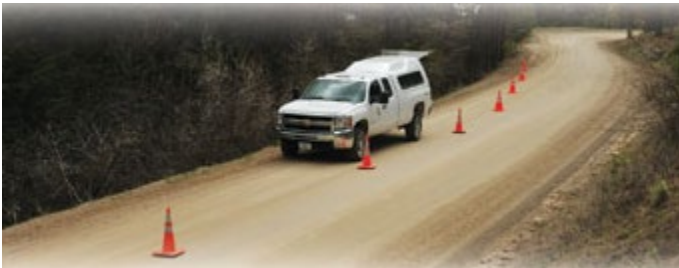
Figure 7: Traffic Cone Placement as pictured by the USS Forest Service. Surface water staff must only park in the shoulder area and never park to completely block a lane of traffic
