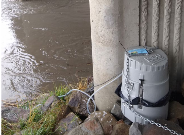
Figure 3: A Teledyne ISCO 6712 portable sampler secured in the field
