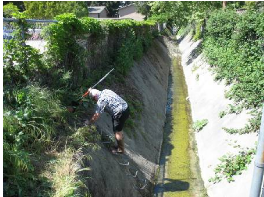
Dublin Storm Drain MCC010
