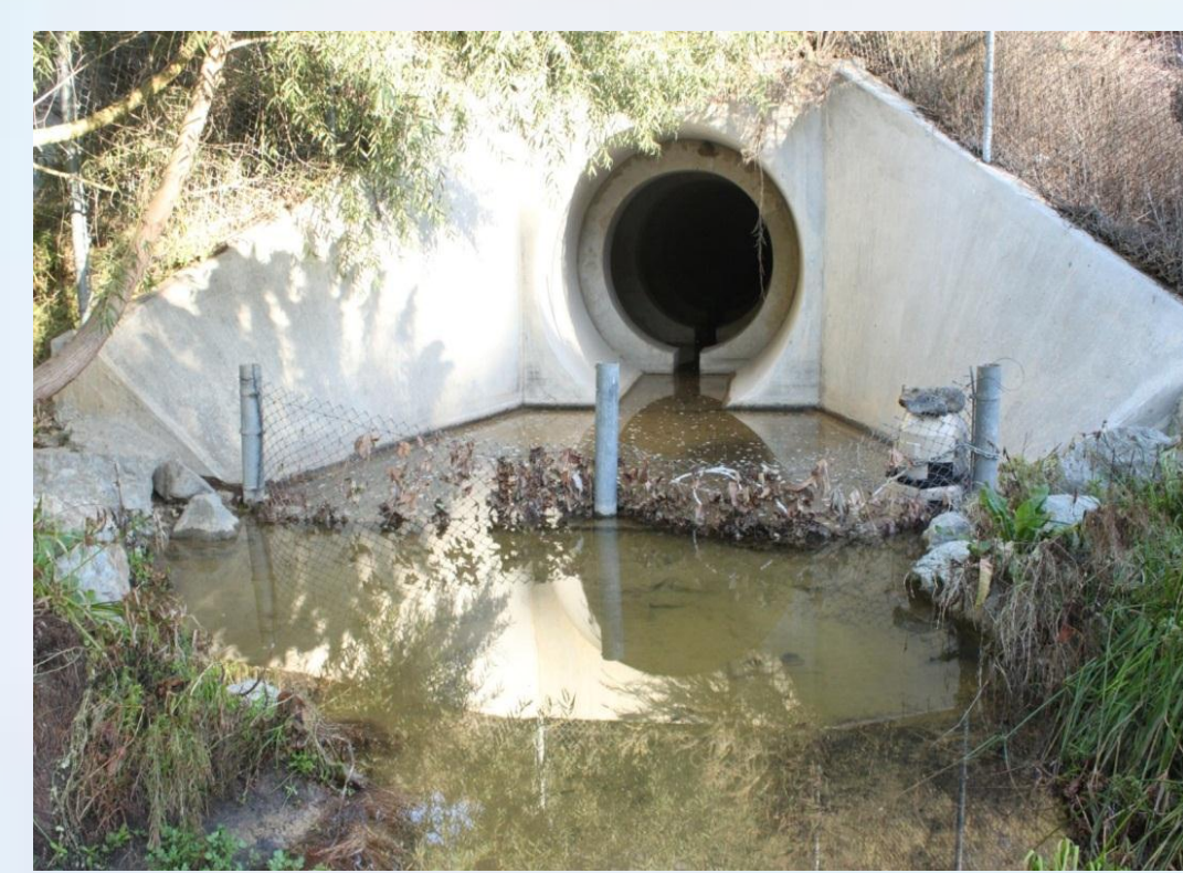
Figure 1. Storm drain entering wetland
