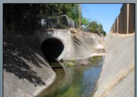
Figure 3. Stormdrain outfall in Dublin, CA (San Francisco Bay Area).
