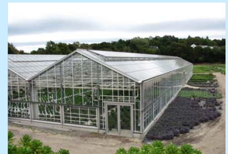
Greenhouse (enclosed space) from Link4
