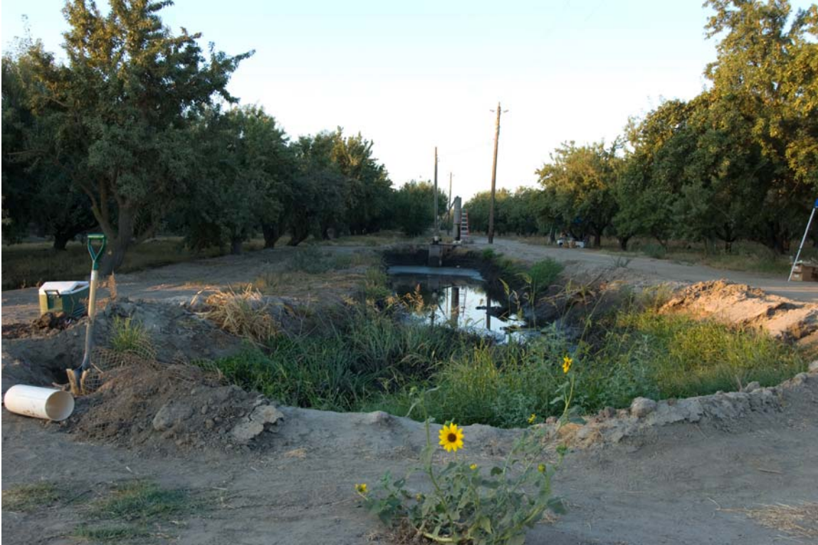
Figure 3. Sediment retention basin
